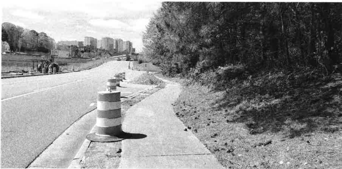
Photograph #10- Interstate North Trail- View of existing trail along Interstate North Parkway SE where anticipated short-term closures of the trail are located. Photographer facing west.
