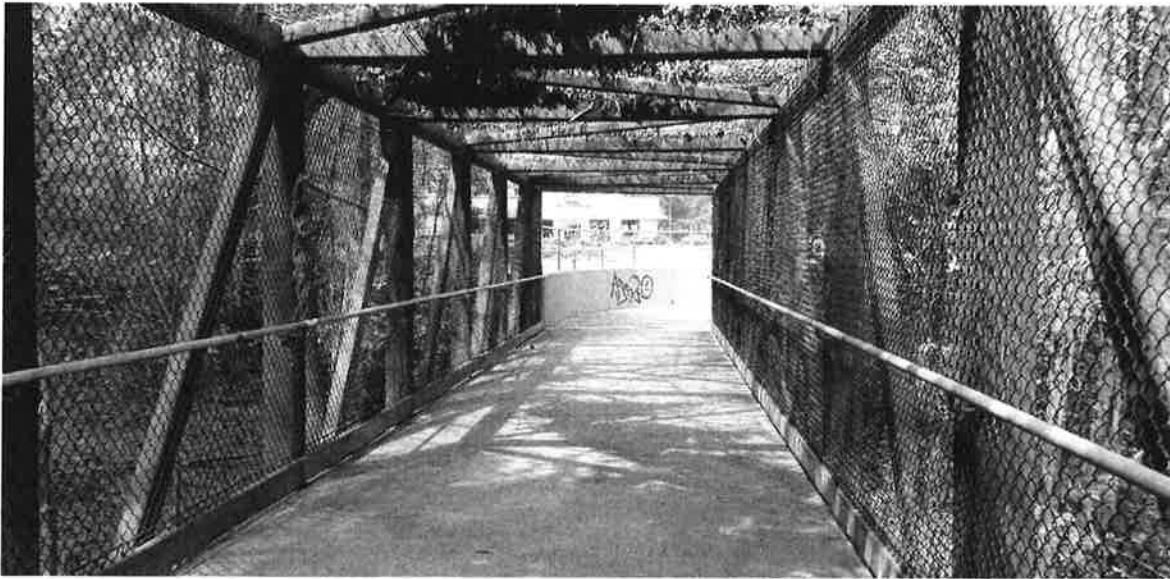
Photograph #6- Mountain-to-River Trail- View of existing trail over I-285, adjacent to Cumberland Blvd SE where proposed express lanes are to be constructed over the trail. Photographer facing west.
