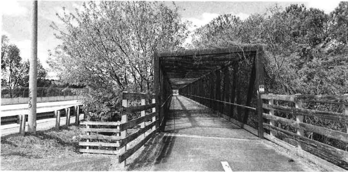
Photograph #7- Silver Comet Cumberland Connector- View of existing trail at Mt. Wilkinson Parkway where proposed express lanes are to be constructed under the trail. Photographer facing west.
